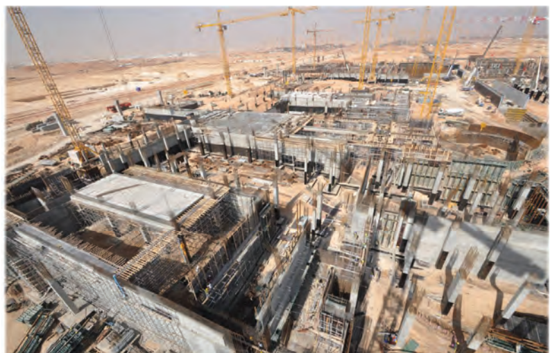
Construction in progress
