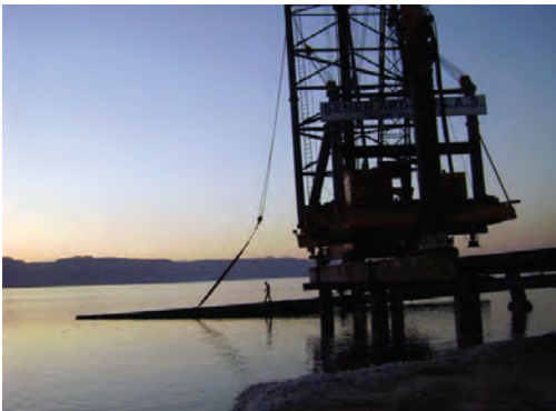
Piles being eased into the water then tugged to their location and crane-lifted into position
