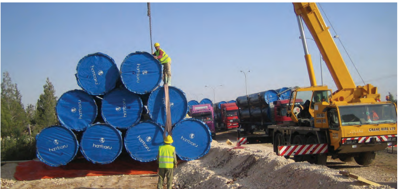
Unloading first pipe shipment
