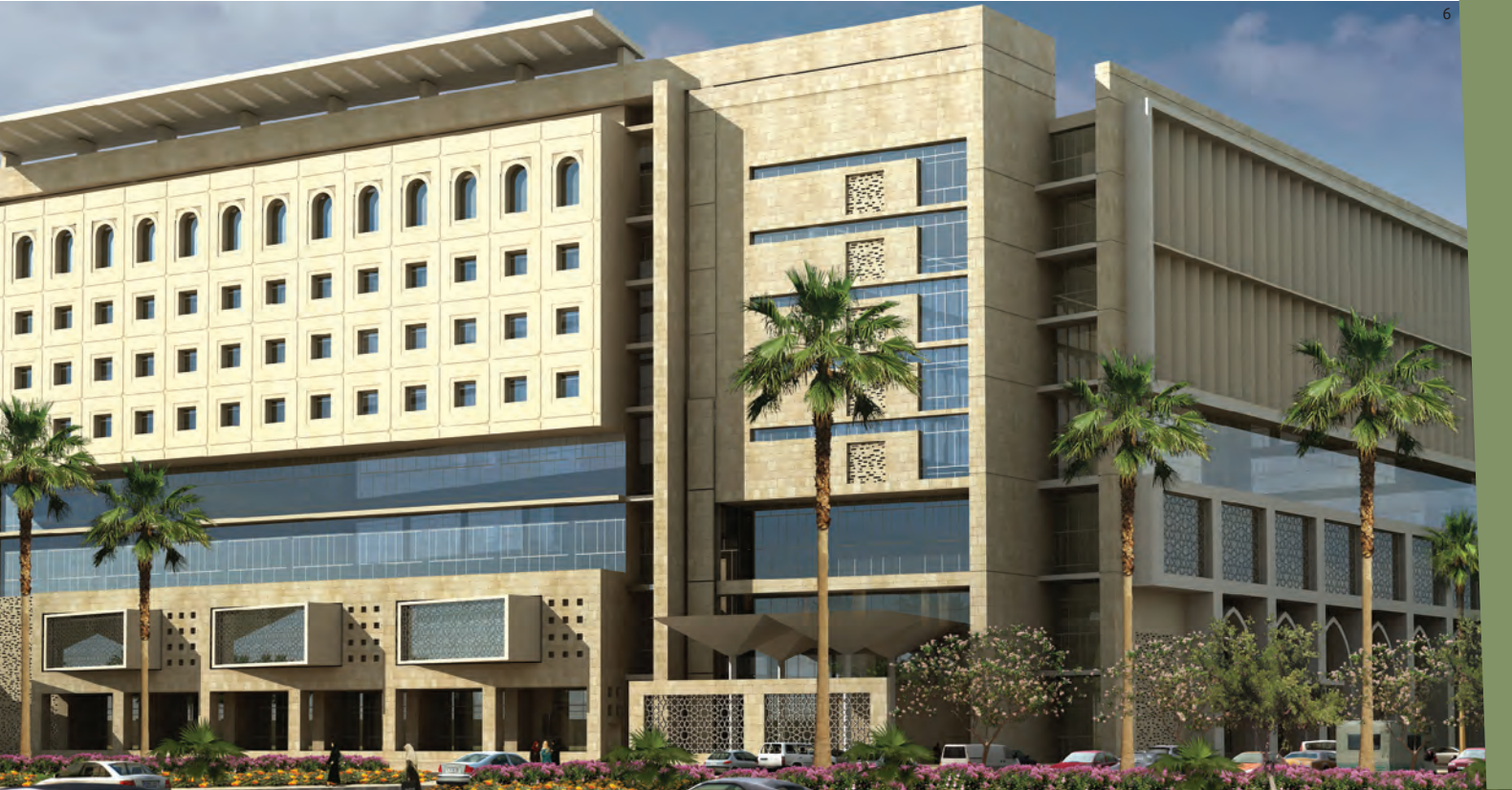
5 Medical Center southern view. In the foreground, the covered walkway to the APM Station connecting the Medical Center to the Health Sciences Campus and the Emergency Room access ramp visible under the atrium podium
