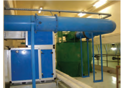
Pneumatic solid waste collection-compaction station
