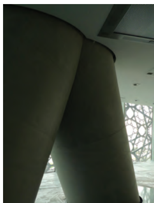
Bottom The tower's circular reinforced concrete 1.7-m diagrid columns, metal decking and reinforced concrete slabs structure and double cladding facade
