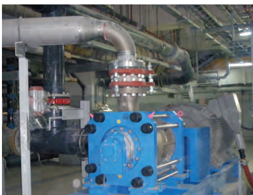
RO cartridge filtration and pressure pump
